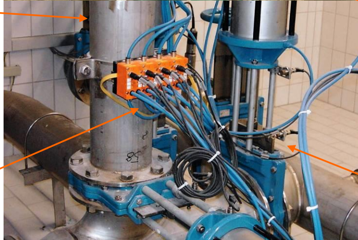
Leakage monitoring with capacitive level sensor e.g. LI5141
